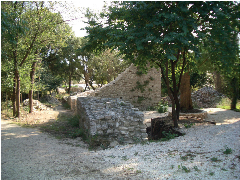
Fig. 1.2 View of the restored western defences (Tower 1). Courtesy of the Butrint Foundation
